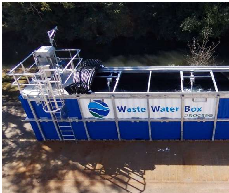
Figure 16 | Ci-dessus | Station conteneur Wastewaterbox, © Cohin environnement
